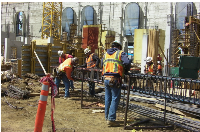
Instead of having ironworkers bend to tie rebar, the work is raised to their comfort zones. Courtesy, Occupational Health Branch, CDPH
